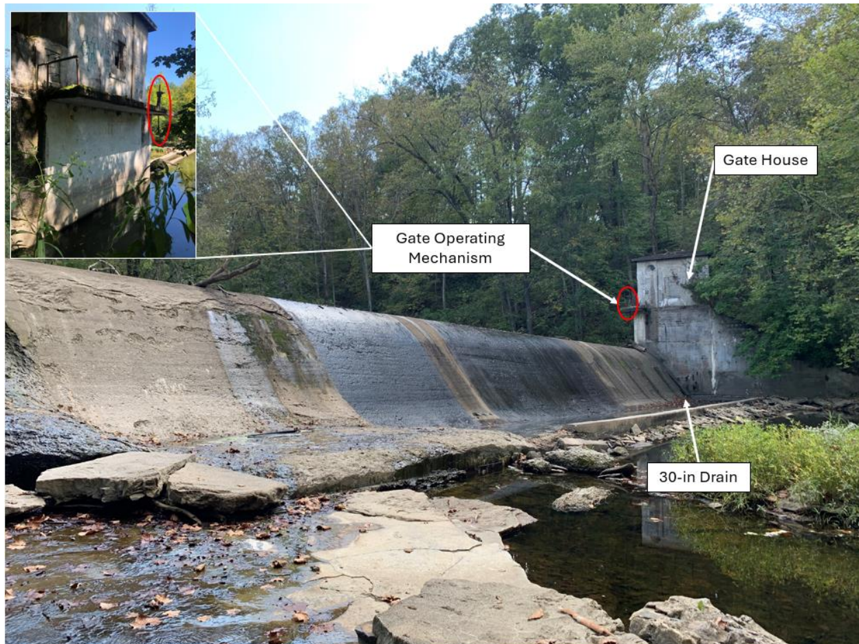
Figure 2-2. Cloverlick Creek Dam looking upstream
