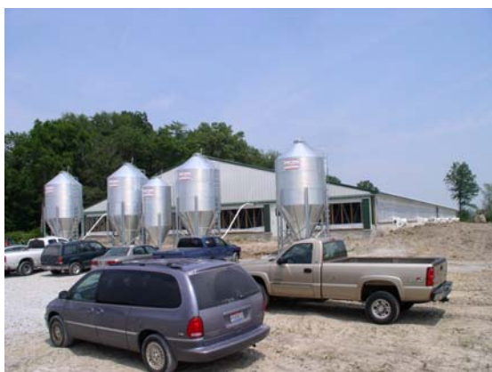
Figure 2-15. This facility in the Lower Dodson Creek watershed in Highland County houses 2200 finish hogs.
