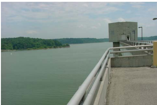
Intake at Harsha Lake
