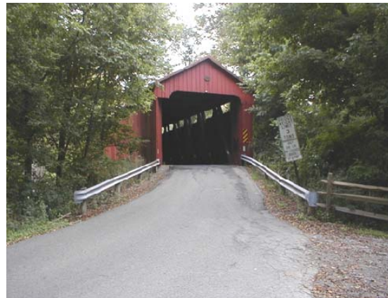
Covered bridge in Clermont County
