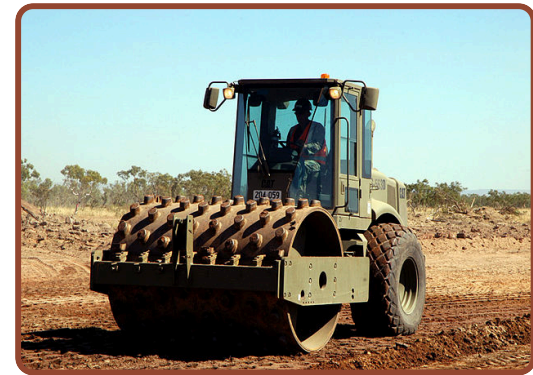
Sheepsfoot roller used for soil compaction
