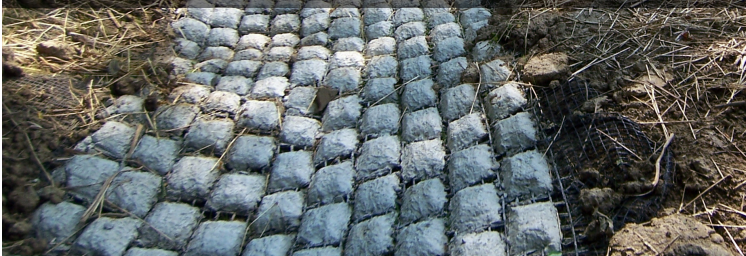
Alternative geogrid product used in a concentrated water channel.
