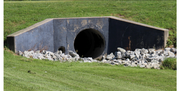
Type C rip-rap used near large culvert outlet
