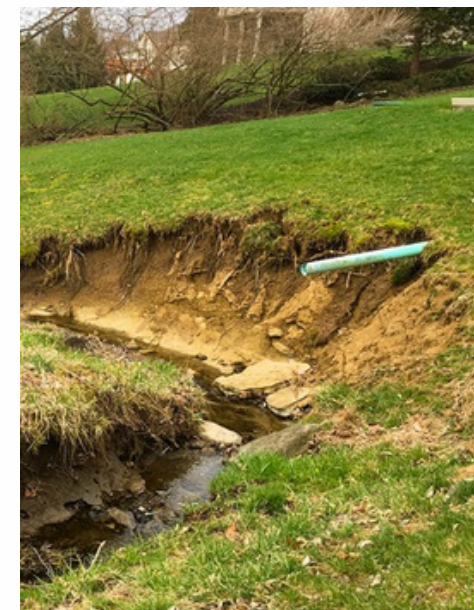
Photo above and below show bank erosion along stream.
