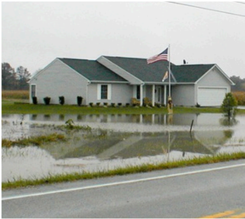
House with poor front yard drainage that is actively flooding.
