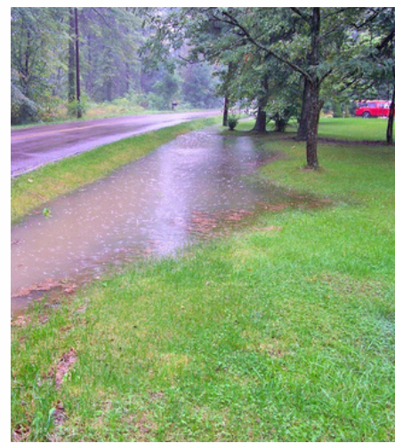
Flooding in a stormwater ditch.
