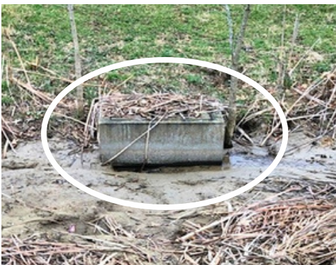
Both pictures showcase non-functional basin outlets. Sediment covering the outlet can slow water exiting the basin
