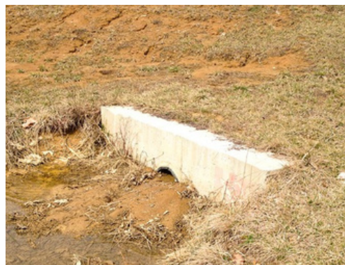
Both pictures showcase non-functional basin outlets. Sediment covering the outlet can slow water exiting the basin
