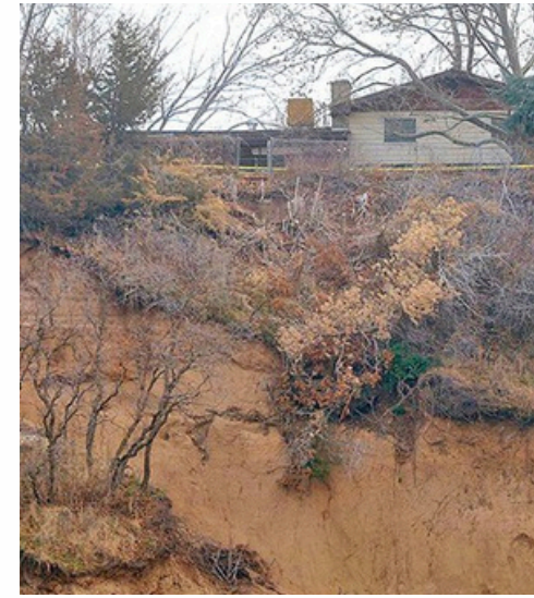
A steep bare hillside has high risk of landslides.
