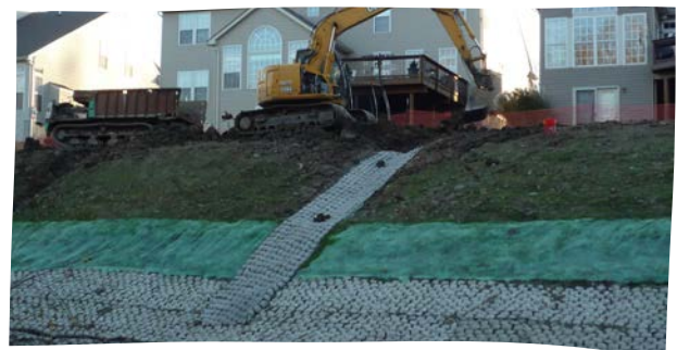
Application of revetment
