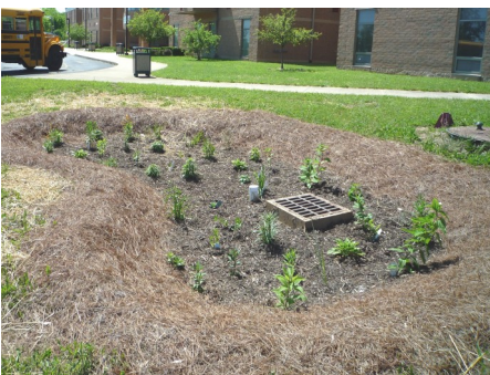
Using catch basin as garden overflow
