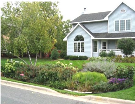
Curb cut capturing street runoff
