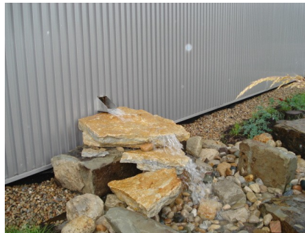
Downspout waterfall flowing to garden
