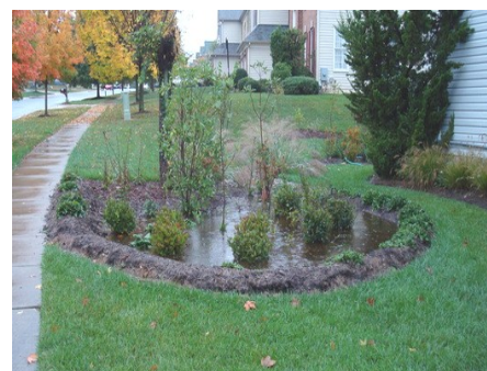
Rain garden capturing sidewalk runoff
