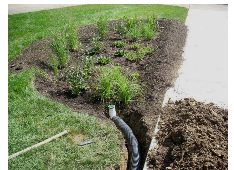
Installing underdrain with standpipe overflow
