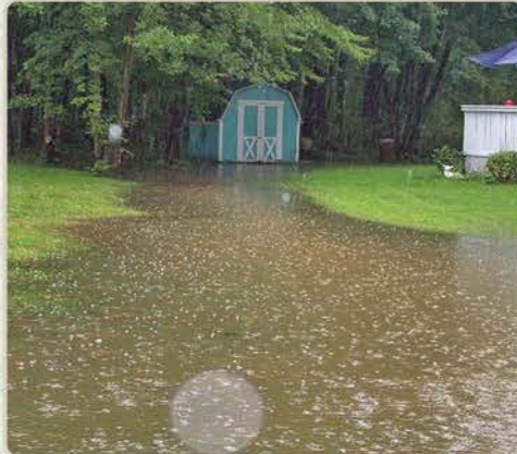
Shed built in a drainage way
