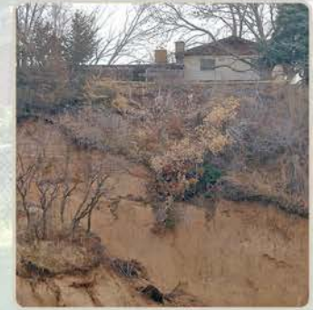
A steep, bare hillside has high risk of landslides.
