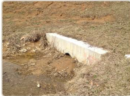
Both pictures showcase non-functional basin outlets. Sediment covering the outlet can slow water exiting the basin
