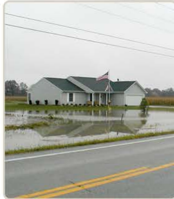
House with poor drainage.
