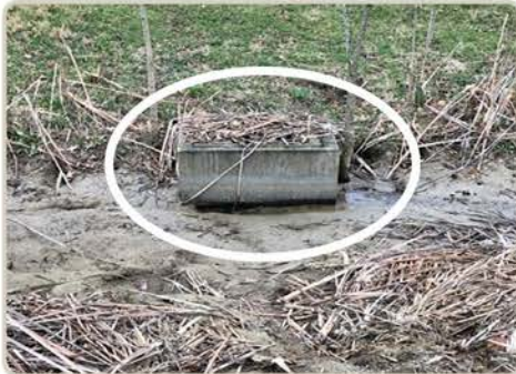
Both pictures showcase non-functional basin outlets. Sediment covering the outlet can slow water exiting the basin
