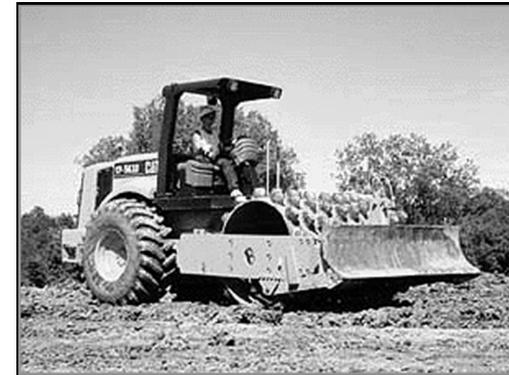
Sheepsfoot roller used for soil compaction
