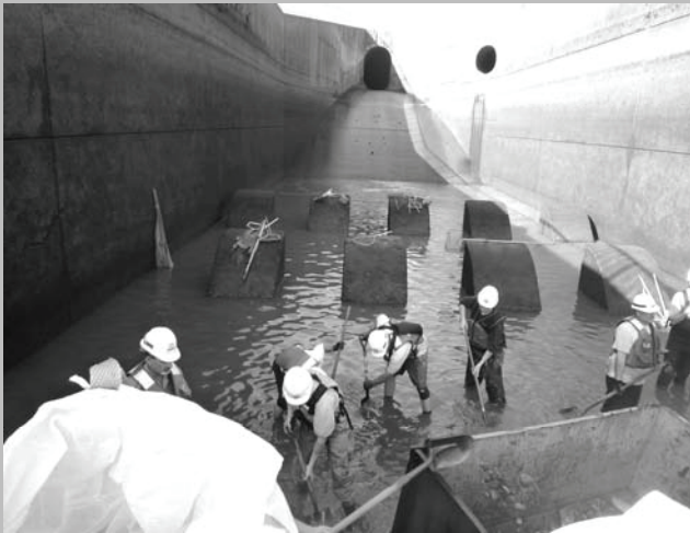
Crew working in stilling basin with lake outlet in background
