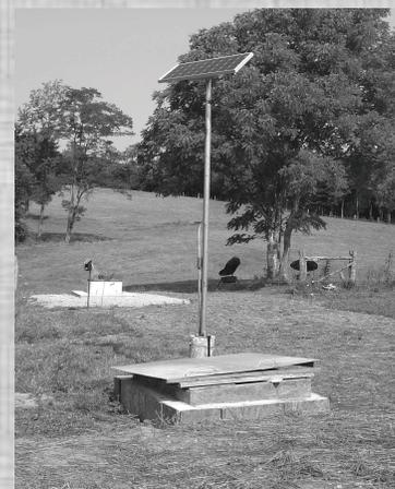
Livestock watering system with spring development and solar powered pump
