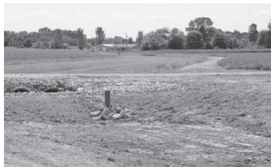
Nearly completed detention structure with planted gravel bed (unmowed) in background.
