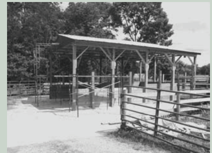
Covered waste storage facility under construction at Cincinnati Nature Center
